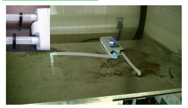
Tighten the handy clamps with a pliers to secure the tubing on the IceZone<sup>®</sup> Unit.
